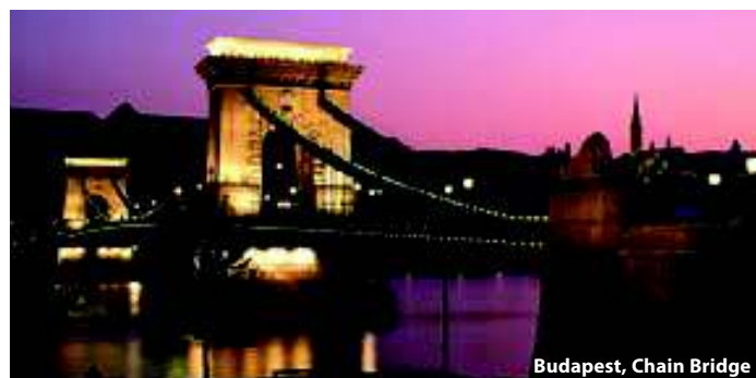
Budapest, Chain Bridge
